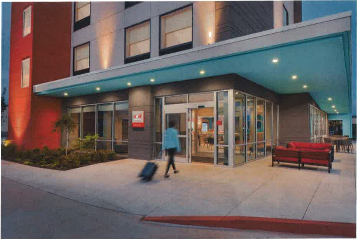
Front entrance with storefront glazing and outdoor seating
