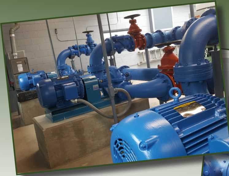
Pumps, motors, and piping in one of the Village's rehabilitated pumping stations.
