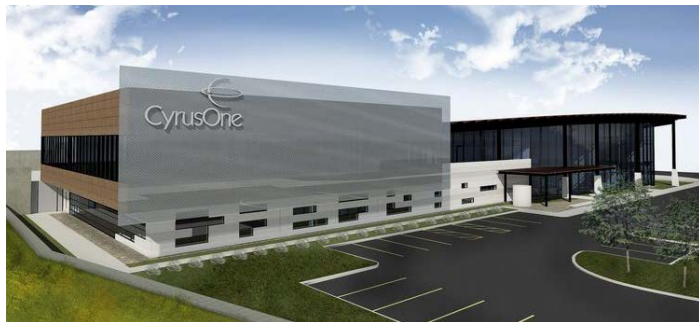
CyrusOne Data Center Westover Hills, TX
