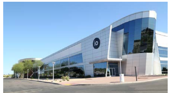
IO Data Center Phoenix, AZ
