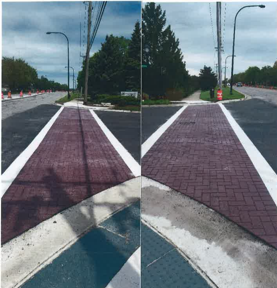
Decorative crosswalk installation in Elk Grove Village - 2021
