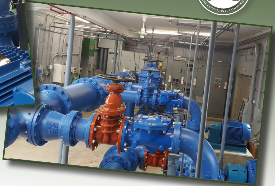
Pumps, motors, and piping in one of the Village's rehabilitated pumping stations.
