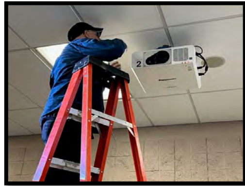
EGTV Technician Mike Meranda installs new projectors in Room E.
