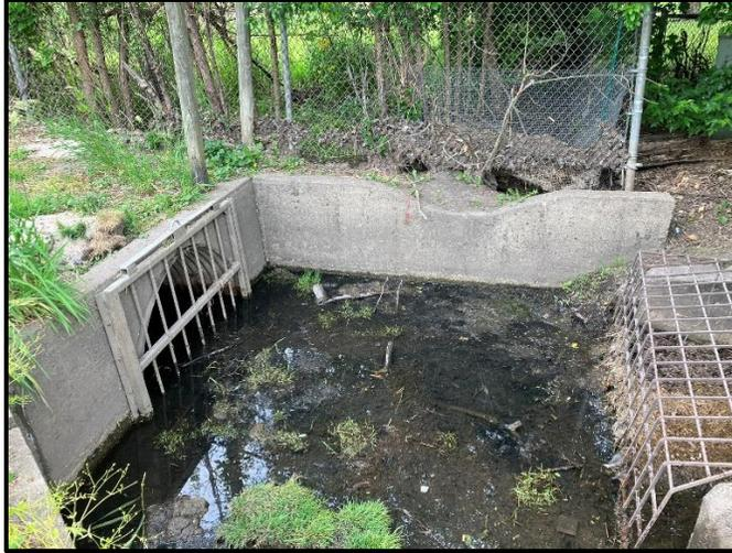
*Figure 1: Location No. 1 for Removal of Existing Structures showing the retaining wall and grating*
