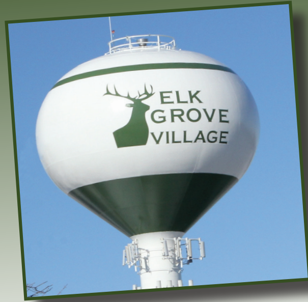
Elk Grove Village water tower design selected as the winner of the Illinois Section AWWA 2014 Tank Photo Contest.
