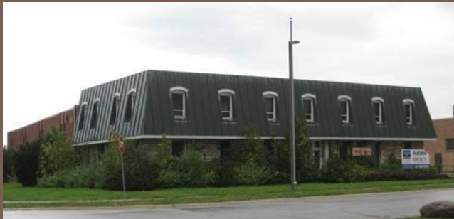
Overgrown & Unkempt Vegetation
