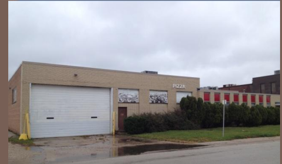
On-Street Docks Broken Windows
