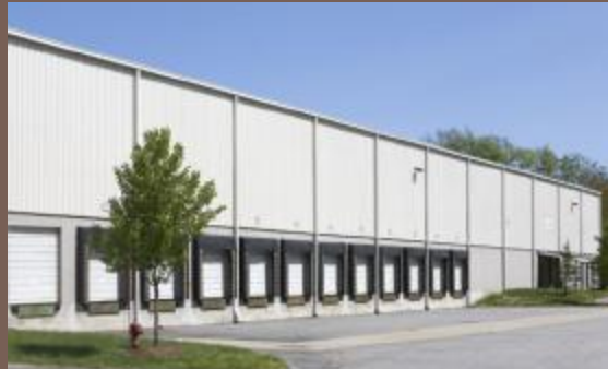
On-Street Loading Docks
