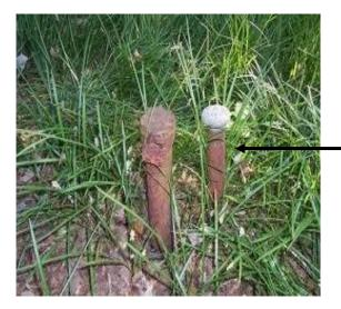
These pipes indicate an existing underground storage tank remains on the property.
