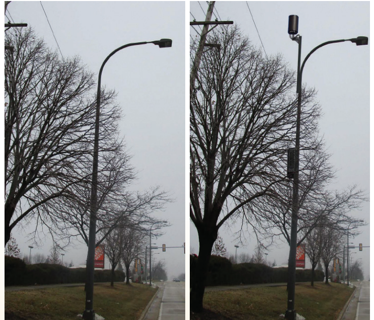
Existing Light Pole
