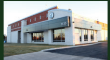
Public Works Biesterfield Facility: 1635 Biesterfield Road
